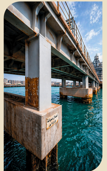
Steel and concrete infrastructure protected by acrylic-based coatings derived from industrial byproducts.
