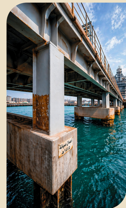
Steel and concrete infrastructure protected by acrylic-based coatings derived from industrial byproducts.
